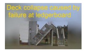
Is your deck properly attached to the building? It's not always possible to know for sure, but today I'll discuss a few different ways of attaching a deck to a building. The piece of wood that connects a deck to a building is called the **ledger**, or **ledger board**. I'll be using this term repeatedly.
