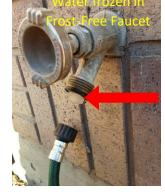
When a frost-free bib cracks during the winter, you may not even realize it until spring. When you turn that faucet on to water the lawn, pressurized water enters the cracked valve tube, and exits into the
